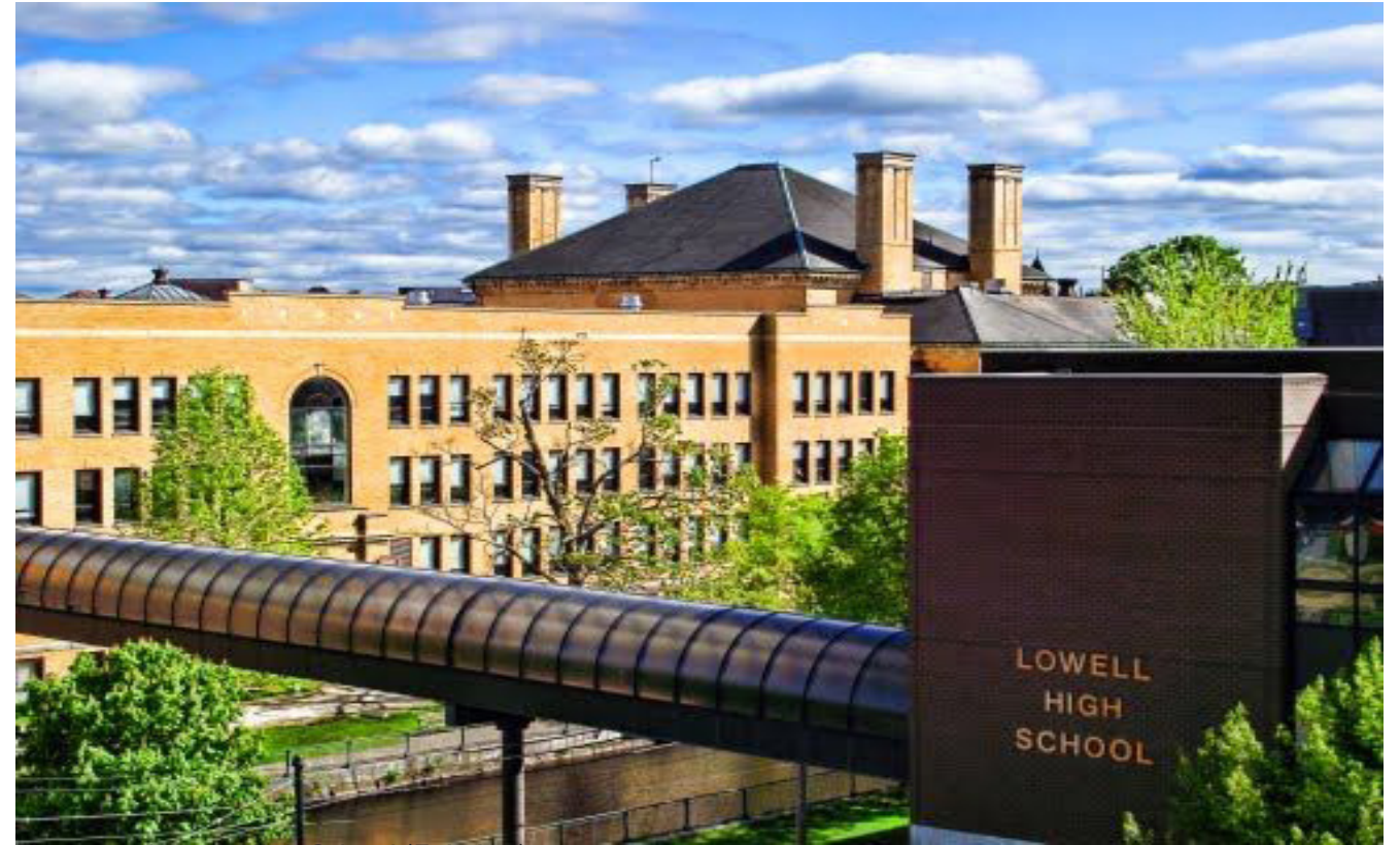
Figure 01. Lowell High School (Existing)
